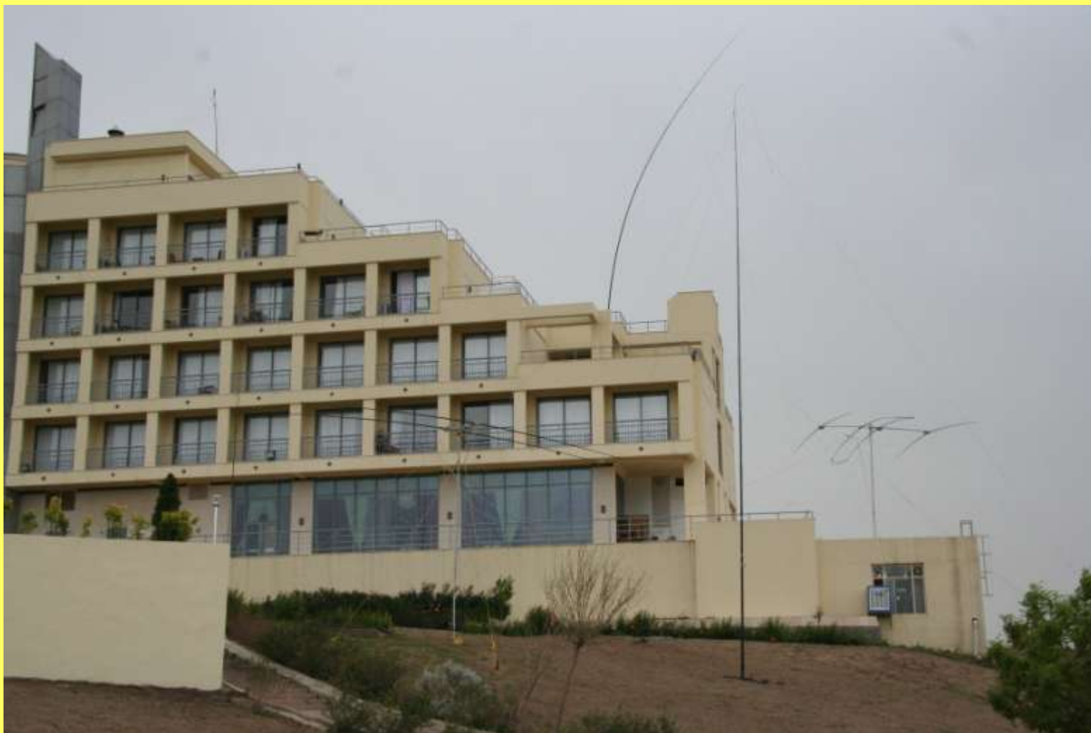
CW antennas, verticals and SteppIR Yagi
