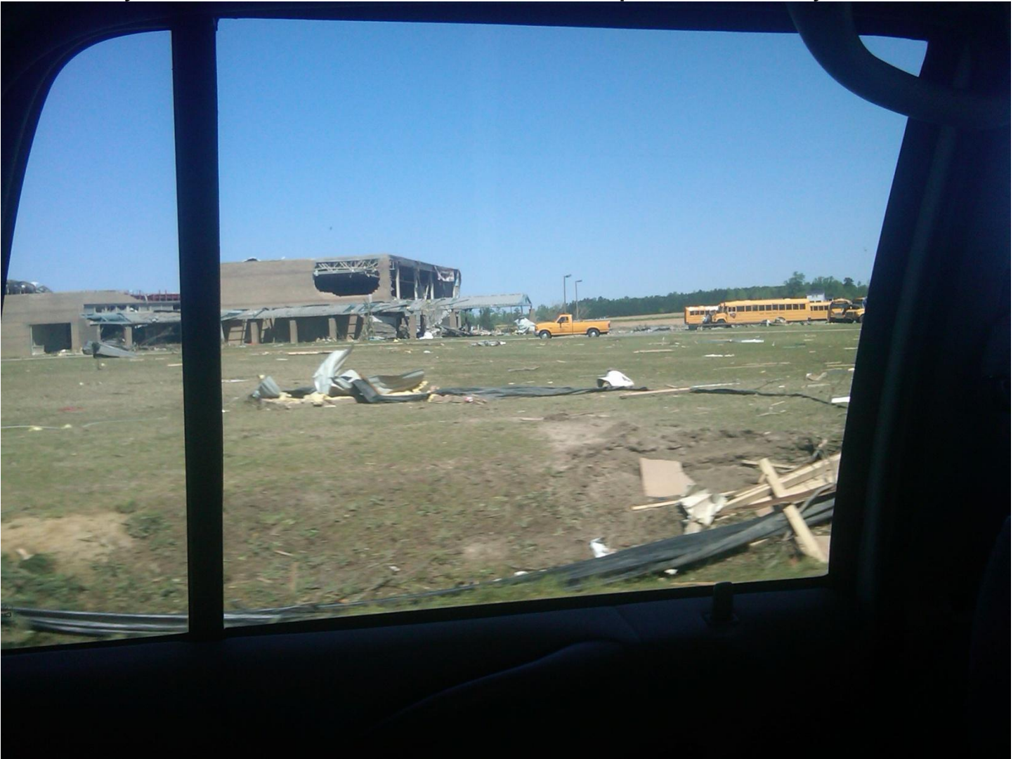
Example of heavy damage to large buildings. Pictured is Green County Middle School.
