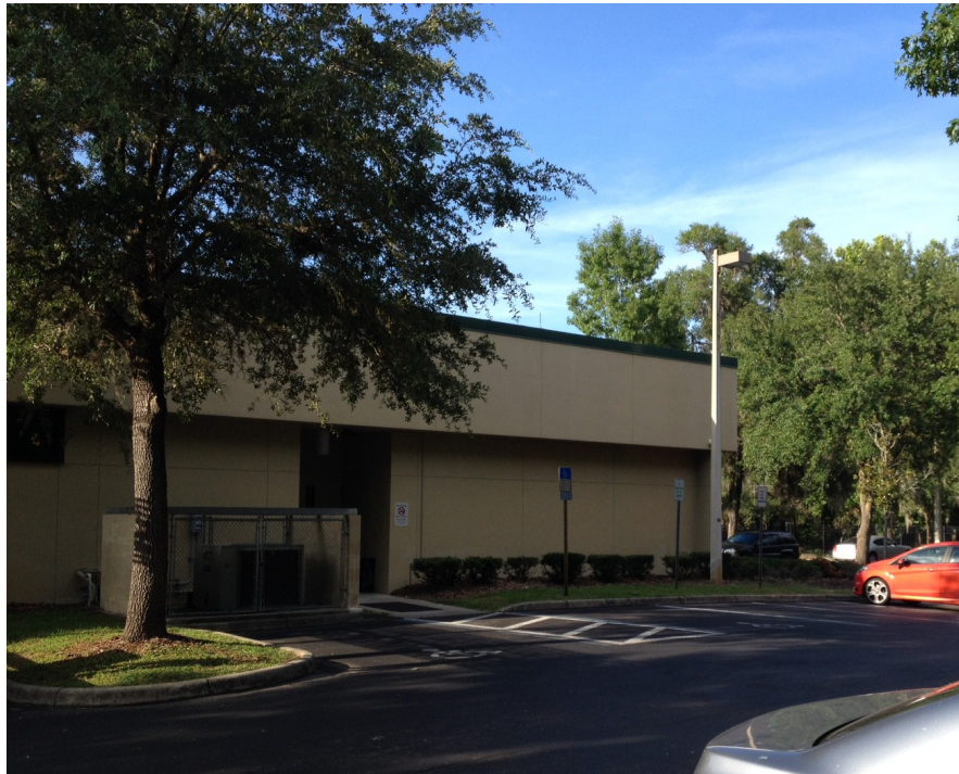
Central light pole for horizontal antenna at the southeast corner of the EOC building.
