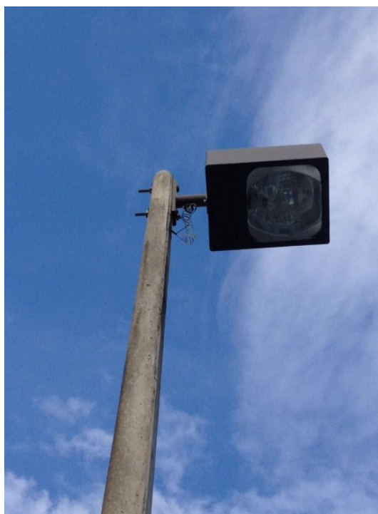
Threaded bolts extant on the EOC light poles.
