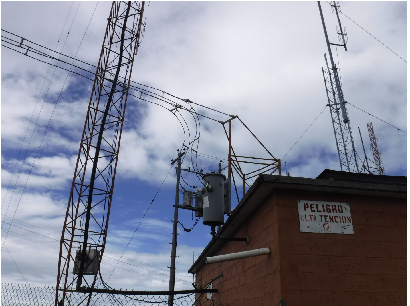
Business end of the Pichincha TX site. AM, FM and SW feed lines
