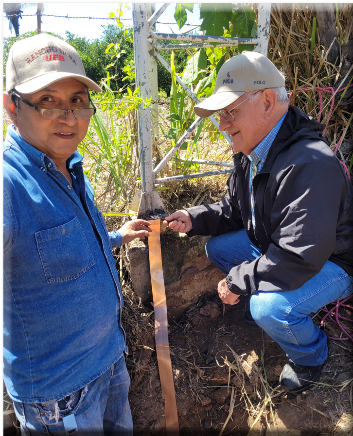
Attaching lightning protection
