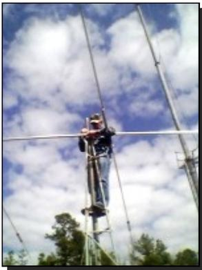
work at the JAARS Center. In the picture here, he is mounting a test beam antenna to be used to show the ability of our team to do emergency communication in a field situation. We do this with portable power only. This will be from a gasoline generator and also from solar panels. Each system will be completely self-contained. The kinds of radio
