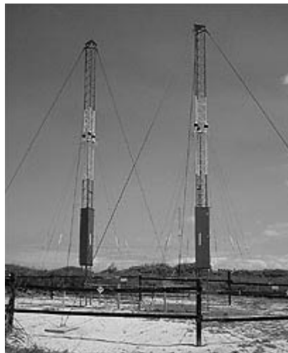
WWVH 15-MHz phased vertical array on the island of Kauai, Hawaii.
