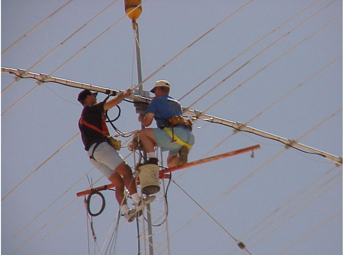
LeRoy, KD7BIA and Paul, G7SLP getting us closer to be loud on the bands. They are here on the 40 m level above the ground.
