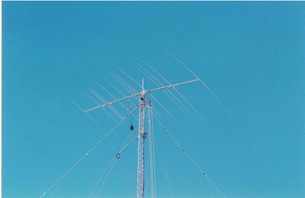
A closer look Coax-baluns for: The 160m Dipole (right of tower under the boom), Delta 80m (left of tower a bit lower) and Double Delta 40m (Lower, two baluns on common horizontal boom, right one close to the tower).
