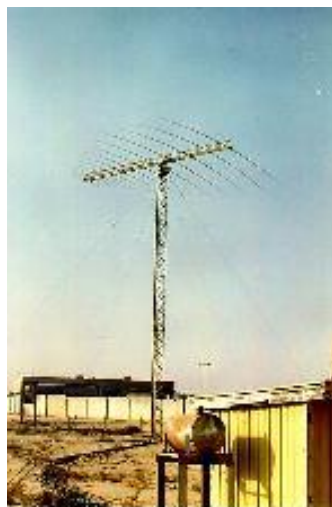
The rotating horizontal log periodic antenna at 60 Ft (18 m). New Shack The yellow hut at front housed the generators that came to use when the mains cable to the shack was cut between Nov. 2002 - Jun 2003. Note the diesel tank.
