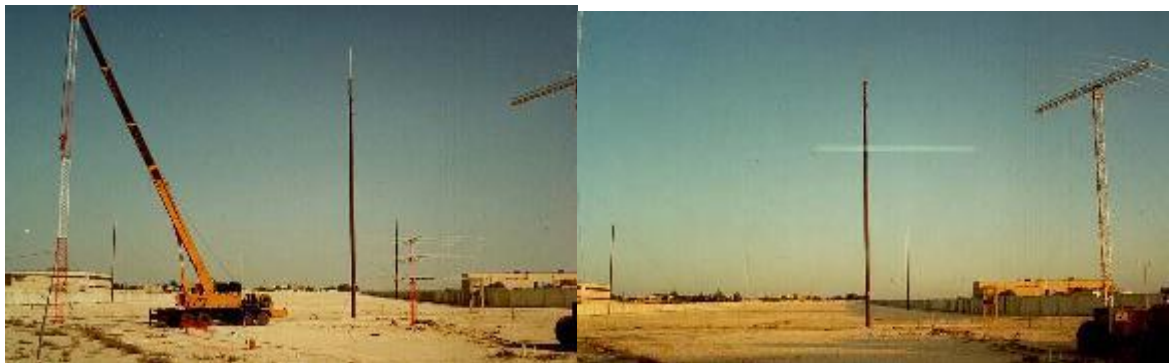
Pole in center is one of the 90-foot poles supporting the famous 850-ft (259m) long Rhombic. The Rhombic was pointed on W0-land, see the Rhombic data. On the right is the log periodic used successfully on 30 and 40 meters.
