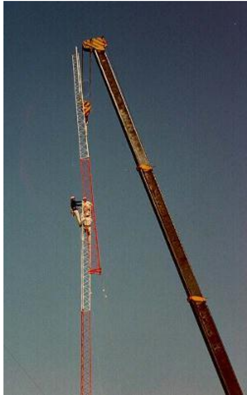
Erecting the 130-foot tower. Riggers are Filipino workers.
