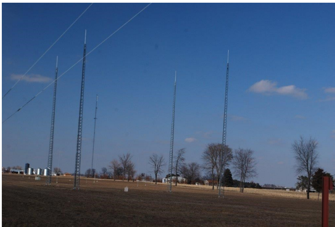
Rather than go with a rhombic for the low bands, Mark decided to go with a 4 square vertical array instead. Mark said putting in the ground radials was the toughest part; especially in the winter time...frozen ground!
