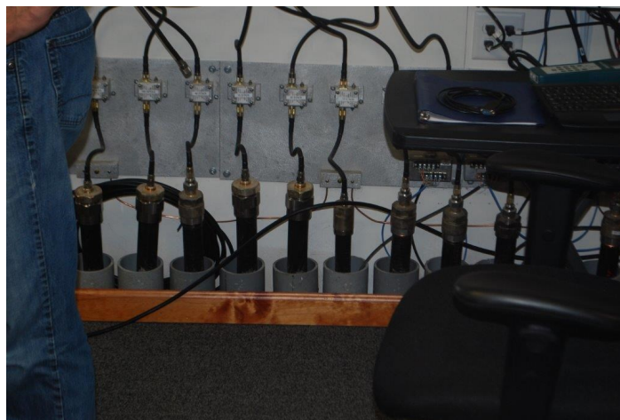
Mark really appreciated Garry, AC9FF's fine presentation on good station grounding, and he wanted to do it right. Notice the polyphasers, coax and grounding plate all at a single point ground.
