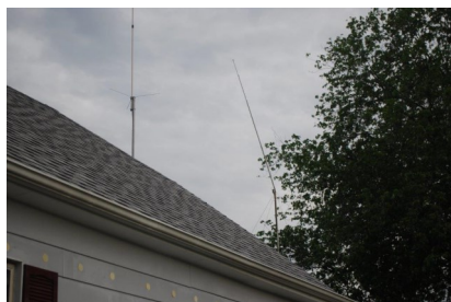
Pictured are John's Comet GP6 dual-band vertical and his 12 meter vertical. Notice that his 12 meter is leaning towards the east. He suffered some antenna damage when the tornado went through the Staunton—Mt. Olive area on Monday May 20th.
