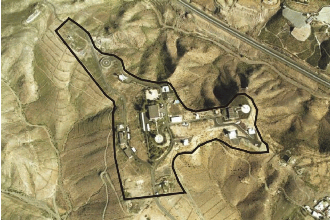
Figure 25: Maspalomas (MSP) Aerial View
