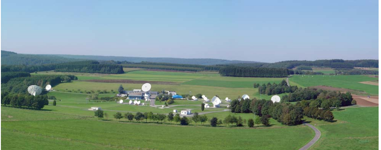
Figure 43: Redu (RED) Aerial View
