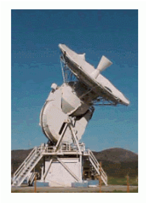
Figure 81: Santiago 9m (AGO-9m) Antenna
