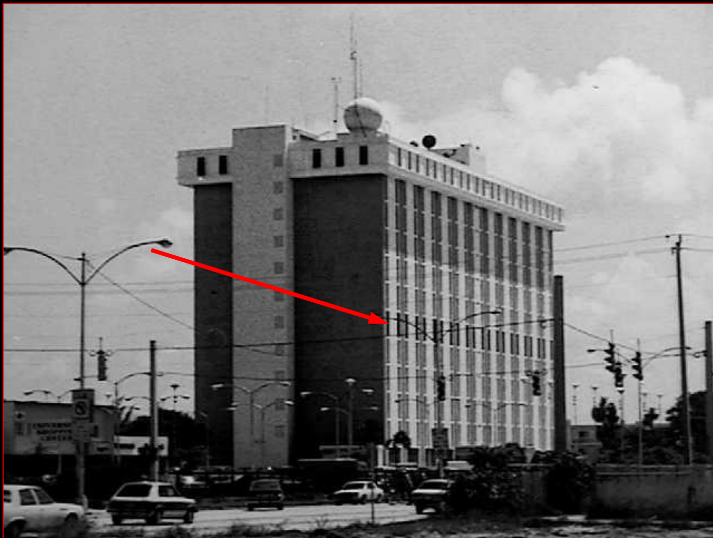
1980 NHC on 6 th Floor of the Gables One Tower Notice it was the only floor with Hurricane shutters!
