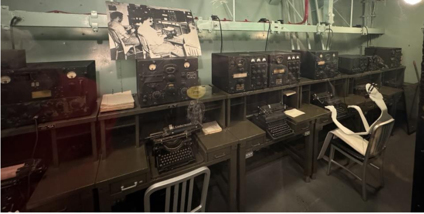
A portion of Radio Central onboard the USS North Carolina (BB-55) in Wilmington, NC.
