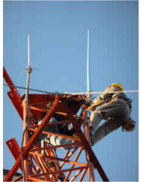
Earl? installing new antenna
