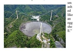
The towers supported the massive instrument platform, which was suspended on cables above the dish. On August 10, an auxiliary cable that helped to support the platform snapped and fell, causing a 100-foot gash in the reflector dish. After an extensive evaluation, NSF announced on November 19 that the damaged radio telescope — in service for nearly 60 years — was beyond
