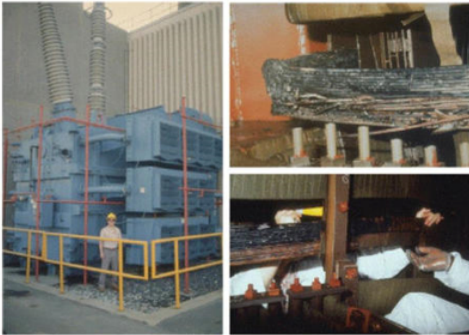
Damage from the March 13, 1989 geomagnetic storm caused by an intense solar flare. (Image credit: NASA/PSE&G)
