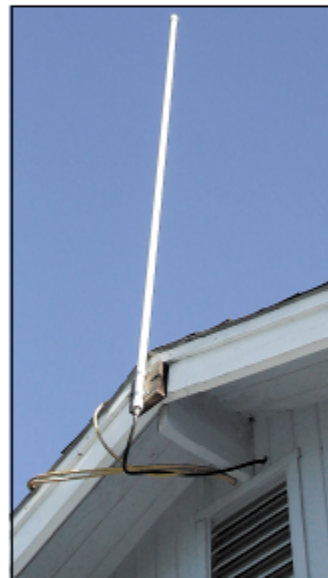
Figure 5—The completed antenna mounted to the roof.
