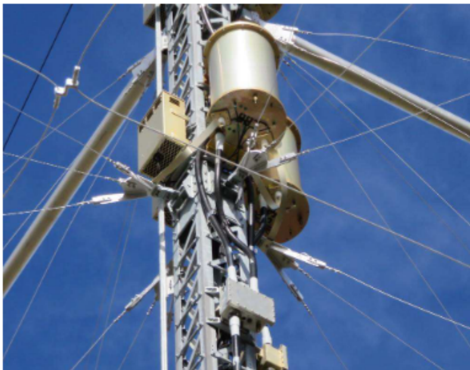
Figure 16 ~ UAF-GI information indicates the balun transformer is the small gray rectangular enclosure in the lower-center directly below the cylindrical antenna matching unit; however, I believe they actually are power splitters and the baluns are inside the Antenna Matching Units. The straps from the antenna matching units to the dipole elements on each side are more easily seen than the previous image. Note also the complex assemblies for joining the bandwidth broadening elements on each of the four sides of the support structure. Image © 2016 W. Reeve
