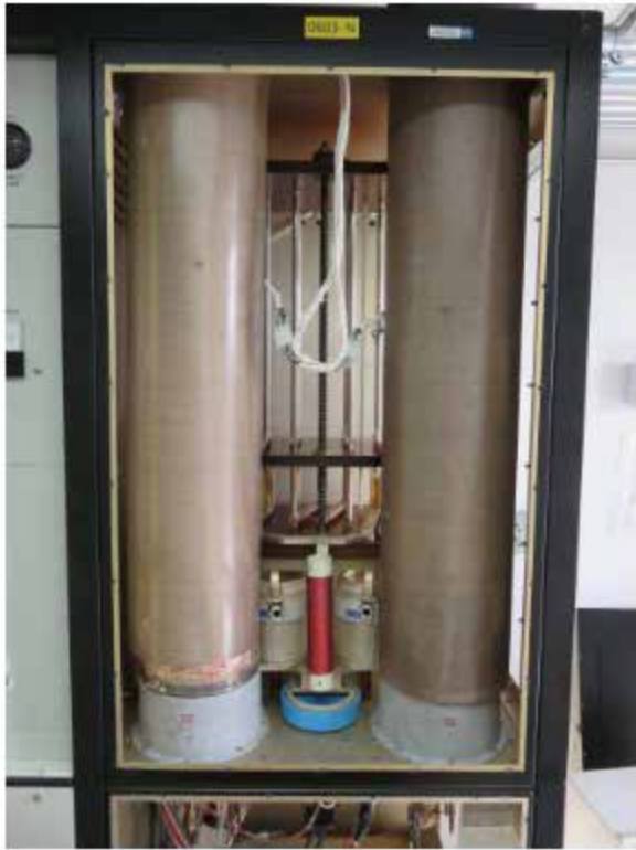
Figure 7 ~ Interior view of a transmitter cabinet. The HAARP transmitters use vacuum tube HPAs (high power amplifiers), and I believe this image shows two of the tubes with what appear to be cooling stacks. Image © 2016 W. Reeve
