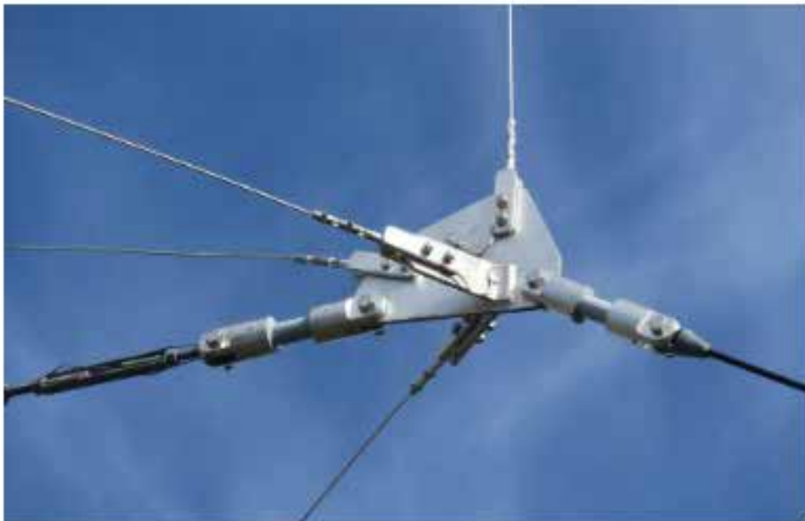
Figure 14 ~ The HAARP antennas are mechanically interlinked for mutual support. This image shows a typical support for four conductive bandwidth broadening elements (silver parts) and two insulated guy wires. It is no surprise the facility cost US taxpayers almost 300 million USD. Image © 2016 W. Reeve
