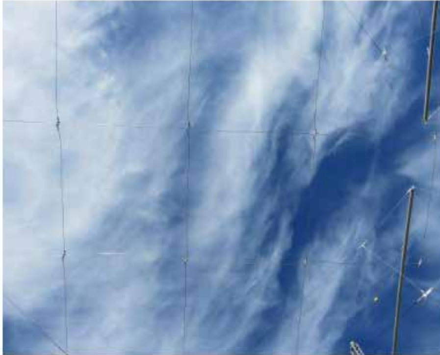
Figure 18 ~ Ground plane (or ground screen) against a background of high thin clouds. The mesh is about 1 m (3 ft), and the wire intersections are held together with special ferrule-type connectors (inset below). Images © 2016 W. Reeve
