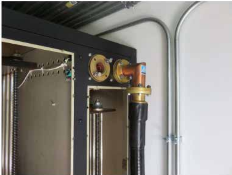
Figure 8 ~ Typical coaxial cable coupling at a transmitter. There are two connectors but only one is used. The coax appears to be 1-1/4 or 1-5/8 in air dielectric corrugated semi-flexible cable; however, I did not see any cable pressurization system manifolds or gauges so the cables may have a foamed polyethylene (PE) dielectric. The jack-screw tuning rods for the matching inductors (or capacitors) are visible in the open cabinet to the left of the cable. Image © 2016 W. Reeve
