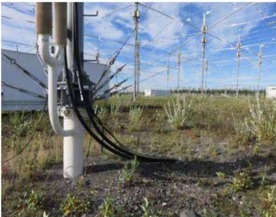
Figure 10 ~ Coaxial cables from the transmitter enclosures to the antennas are direct buried and emerge from the ground near a thermal pile, where they are attached to the tower and rise for connection to the baluns and antenna matching units associated with the crossed-dipoles. Note the numerous guy attachments from adjacent towers. The piles not only support a tower base but also are anchors for adjacent tower guy wires. Image © 2016 W. Reeve
