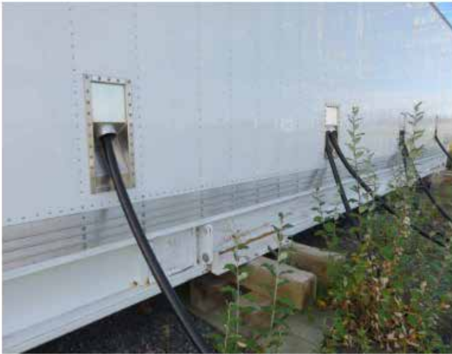
Figure 9 ~ Cable exits at a transmitter enclosure. The stacked timbers underneath the enclosures indicate the enclosures are free-floating and do not have thermal piles for foundation support. Image © 2016 W. Reeve
