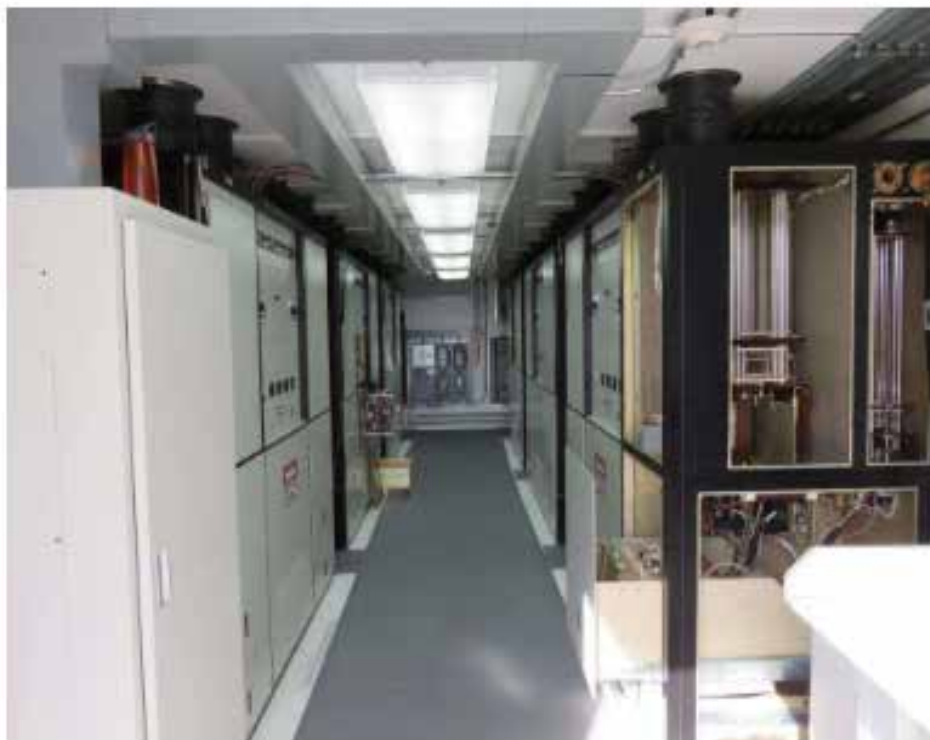
Figure 6 ~ Interior view of a typical transmitter enclosure. A central aisle provides front access to equipment cabinets on either side. On the near-right, one of the transmitter cabinets has been opened for examination. I believe the exposed components in the two upper compartments are motorized tuning inductors or capacitors (or both). Image © 2016 W. Reeve
