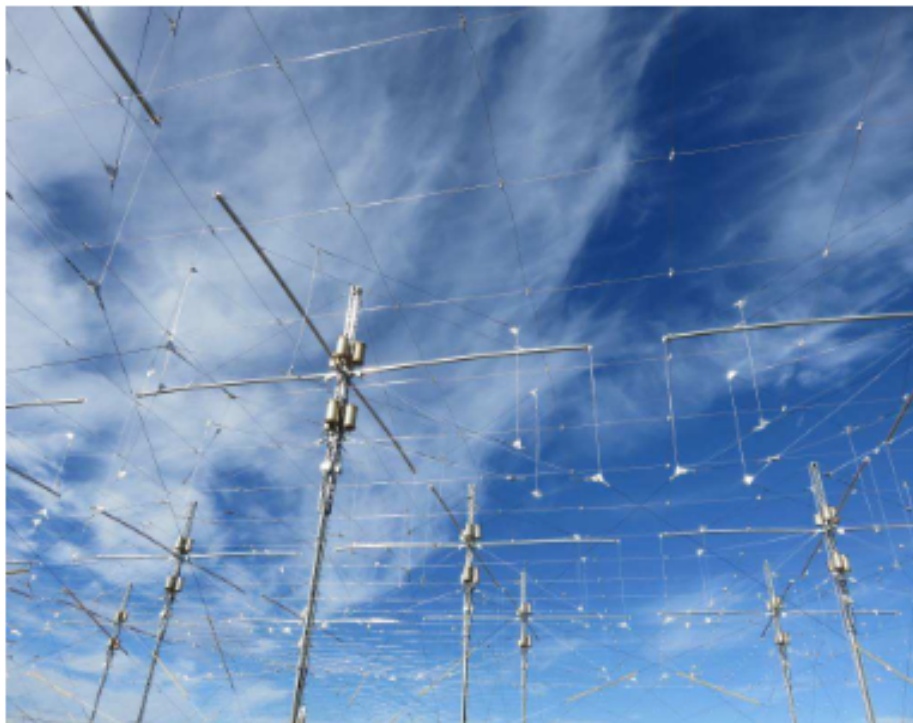
Figure 12 ~ The cobwebs of conductive antenna wires and non-conductive guy wires and messenger strands associated with the antennas and supporting structures are apparent in this image. Seen here are the main crossed-dipole pipe elements near the structure top and bandwidth broadening wire elements, supporting guys, antenna matching units and baluns and the elevated ground plane. It is quite difficult to visually separate them even when standing below. Image © 2016 W. Reeve
