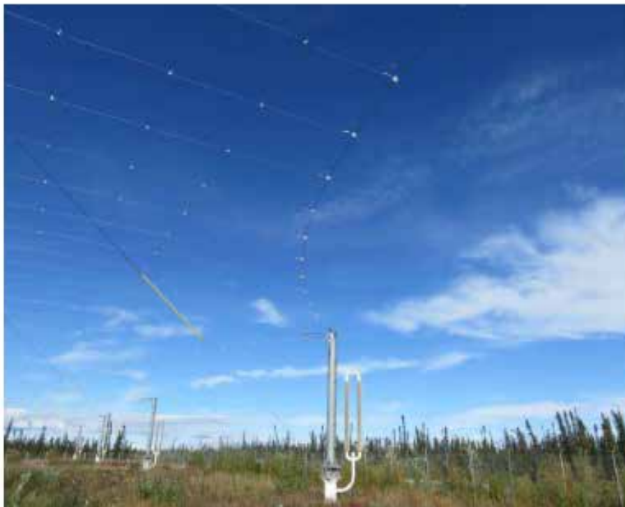
Figure 19 ~ View of one edge of the ground plane against a blue sky. The ground plane extends from the center to left side of the image. It covers a larger area than the antennas. The thermal piles shown here provide support for the ground plane and also are anchors for the antenna support structures. Image © 2016 W. Reeve
