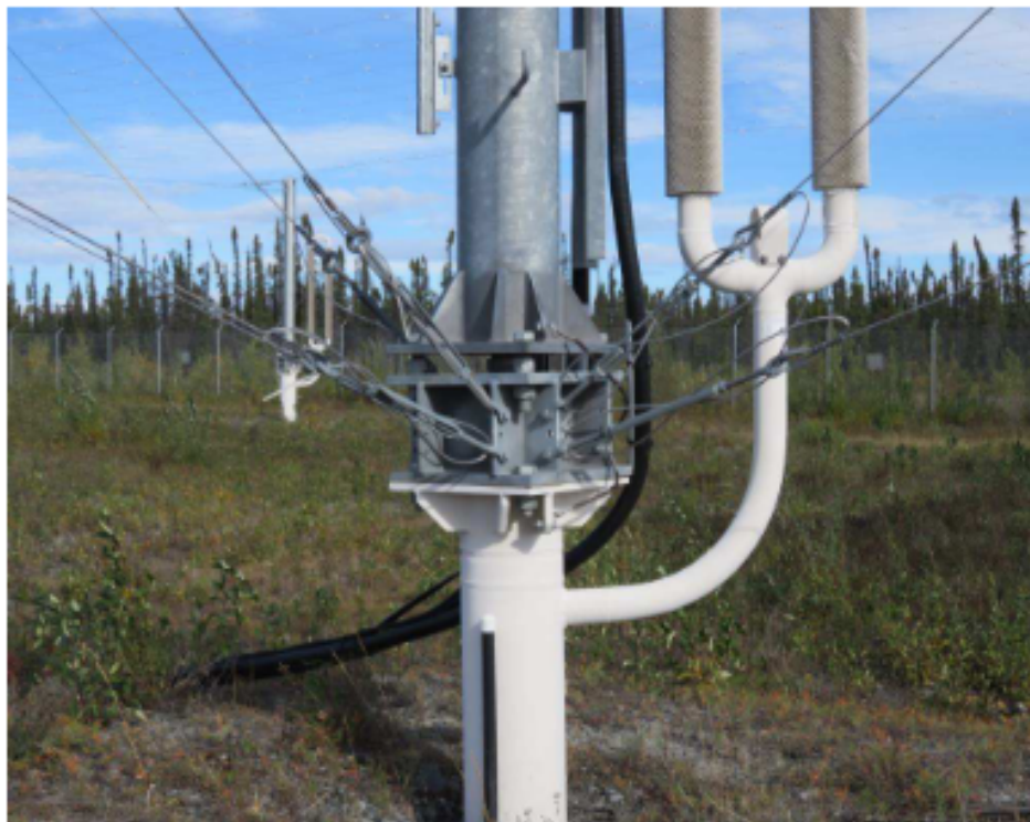
Figure 17 ~ Thermal piles are the white pipes shown here. The larger pipe provides mechanical support for each antenna support structure and keeps the ground frozen year-around. The galvanized steel tower base is mounted directly to the top of the pile and guy wires from adjacent towers connect to it for anchoring; the mechanical loads are symmetrical. The heat absorbing portion of the piles probably is buried a few tens of meters, and the heat is dissipated by the loop to the right. The black tubing behind the pile is the coaxial cable feeding the dipoles. Image © 2016 W. Reeve
