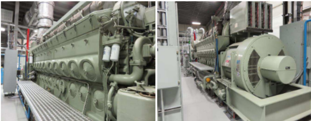
Figure 22 ~ Left : One of the five 4000 hp (3 MW) diesel engines. Right : A 2.6 MW electrical generator. The generators were originally designed for pulsed loading from an OTHR. Images © 2016 W. Reeve
