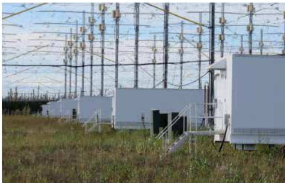
Figure 5 ~ The white transmitter enclosures appear to be modified shipping containers, 40 ft (12 m) long. The green enclosures near the center of this image are step-down power transformers and medium voltage (12.5 kV) sectionalizing terminals that serve two enclosures. Image © 2016 W. Reeve
