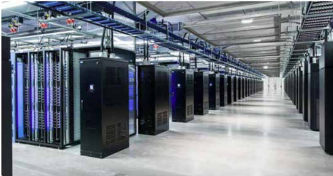
The server room at a Facebook data center | Source: Facebook/Meta
