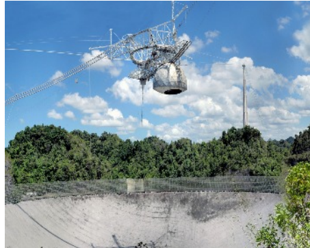
The line feed antenna can be seen pointing downward from the overhead array of equipment.
