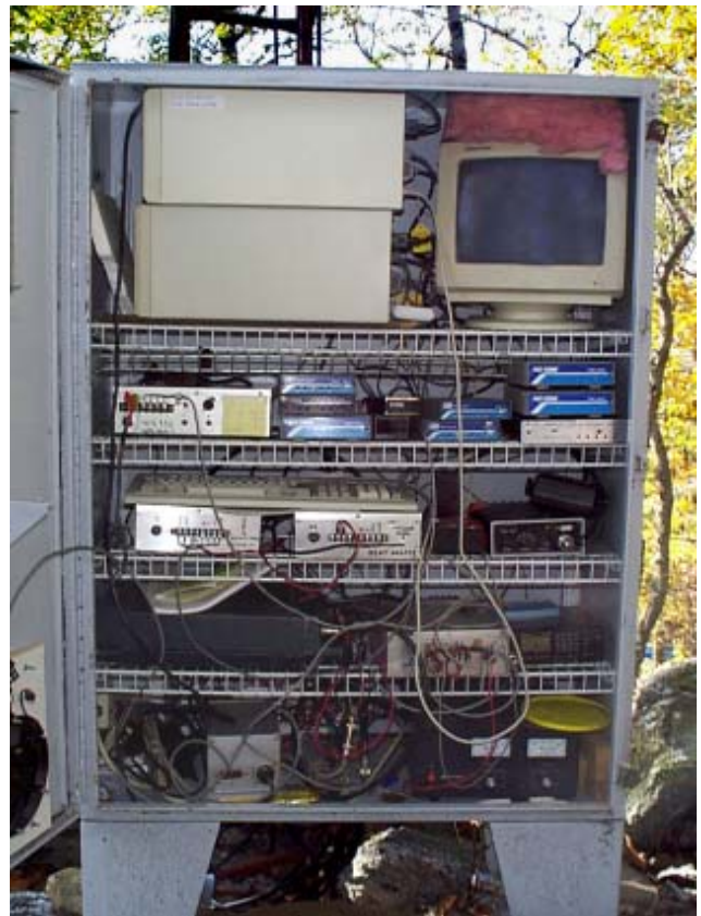
Figure 1: The mountaintop site of the Ramapo Mountain ARC, WA2SNA. This cabinet has AC power and is easily accessible, even in winter. Some node sites aren't as lucky. One of the computers runs the FlexNet node, the other runs NOS. Neither computer is modified for outdoor operation, and both have survived for a few years without problems.
