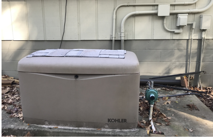
23KW Propane (500 gal) Whole House Generator
