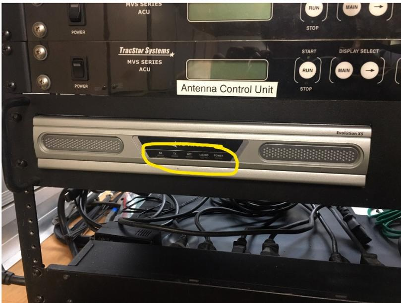
Figure 4-4: Status lights on Modem
