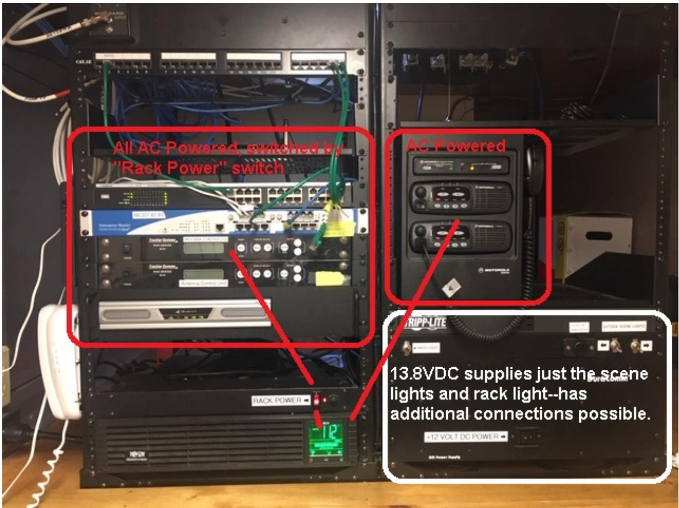
**Figure 2-5.** *Explanation of how power is provided to rack-mounted equipment The items in the left rack are AC powered by the UPS system, through an extension box which has a “Rack Power” On/Off switch. Additional items are directly wired to the UPS, such as the Motorola Repeater. The 13.8VDC power supply in the right lower rack at this time powers ONLY the rack light (very small lamp) and the four large outside “Scene Lights.”*
