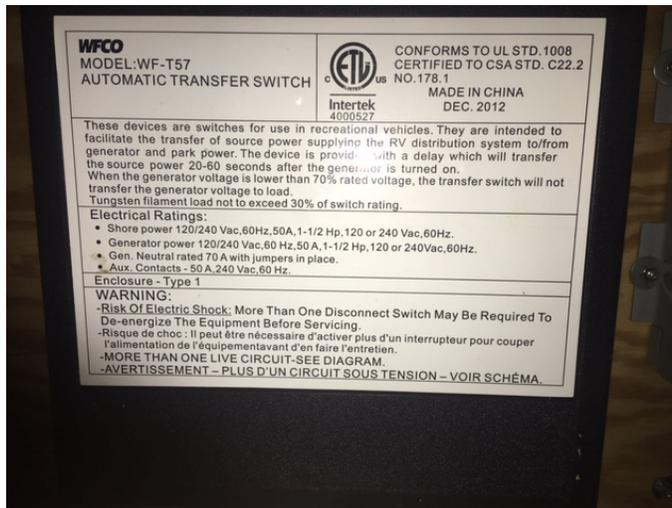
Figure 2-4. Explanatory Placard on the Automatic AC Transfer switch
