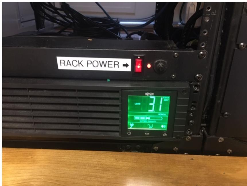
Figure 2-17 UPS and Rack Power ON/OFF Switch
