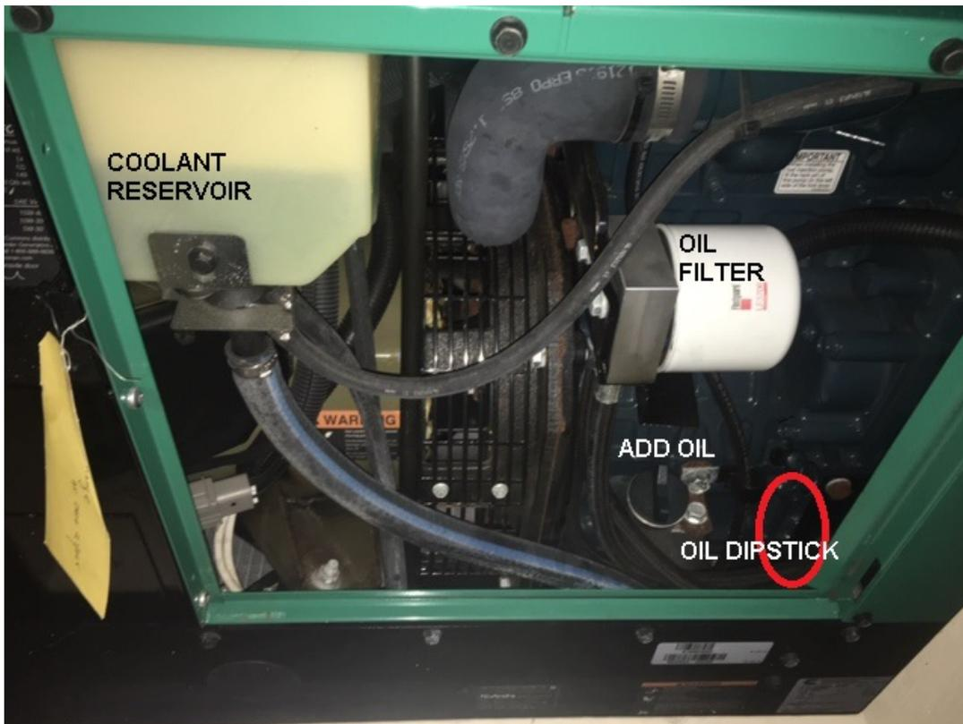
Figure 2-3: *Front of “ledge”, open door and then remove the side access panel of the generator to get this view providing access to the oil dipstick, filter, and coolant reservoir..*
