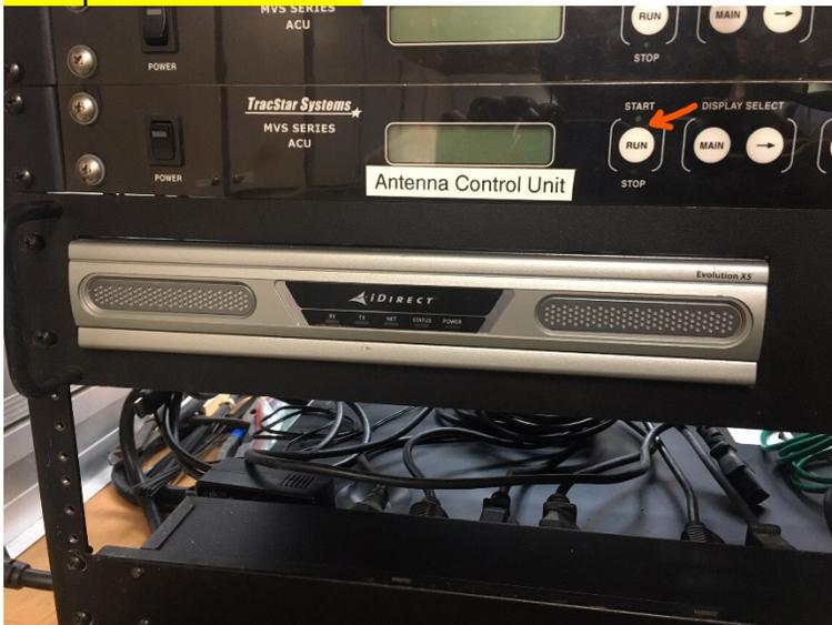
Figure 4-2 Antenna control Unit
