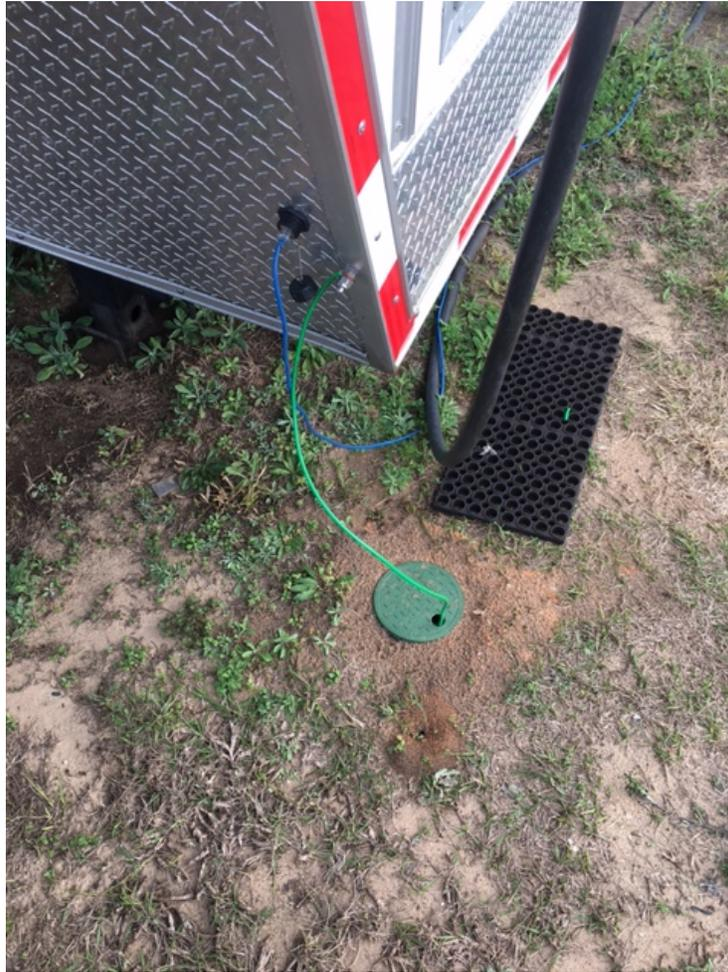
*Wire to buried ground rod (courtesy of Mike Crisler). Note the network connection also in this photo.*
