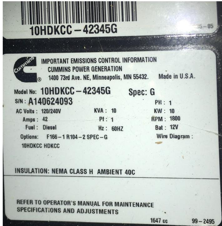
Figure 2-2 Onan Diesel Generator 10-HDKCC Spec G
