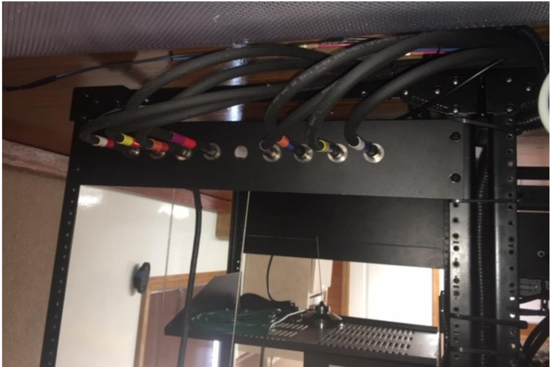
Figure 2-14 Mast Antenna Coax connector terminations on Rack
