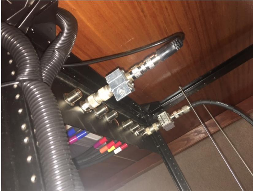
**Figure 2-14** *Lightning Arrester protections at rack. Since this photo, additional lightning arresters have been added.*
