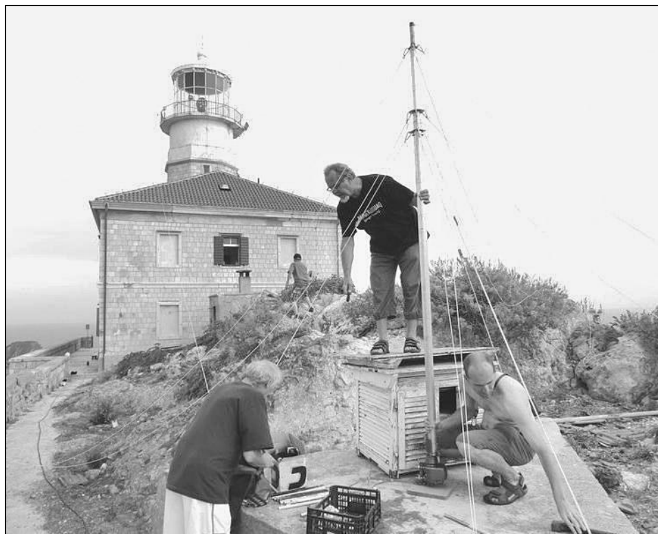
We installed the Spiderbeam antenna, however it was damaged by a storm soon Instalujeme anténu Spiderbeam, bouře nám ji ale brzy důkladně poničila
