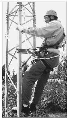
Figure 28.21 — The fall-arrest lanyard is above the climber so that the climber can climb up to it. The fall-arrest and positioning lanyards are then "leapfrogged" so that the climber remains attached to the tower 100 percent of the time. [Steve Morris, K7LXC, photo]
