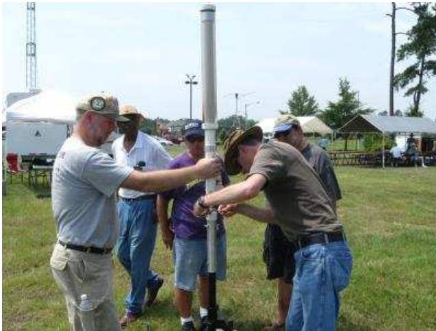
How many does it take to install a Tarheel Antenna for the GOTA station? 2 workers and 3 supervisors!
