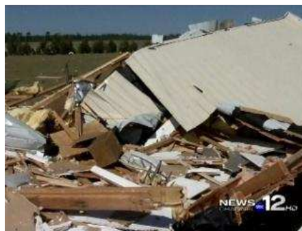
The nearby metal garage was also destroyed along with his Harley.
