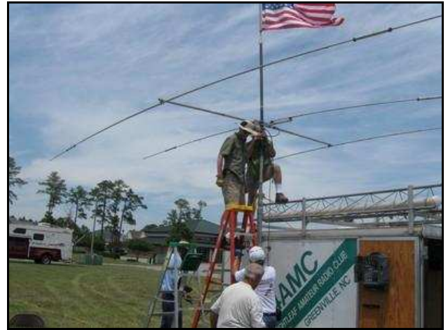
KI4PWX, & W4JNC, installing TA-33 Jr with ground support from WA4MOK, WA4SLC and WB2YFM.
