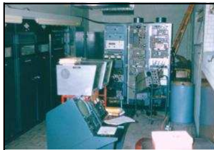
Transmitter control room. Transmitter is on left and the equipment racks on the far wall. Behind the transmitter were big fans for cooling the transmitter. Very noisy and hot!
