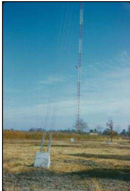
From the tower anchor, you can just see the top of the transmitter building because it was in a hole. They flood when a hurricane comes! Notice the twin guy wires on the anchor.
