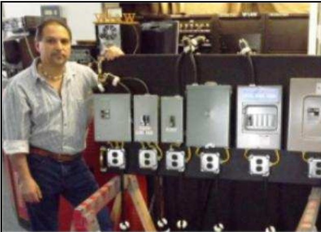
W1AW Manager Joe Carcia, NJ1Q, with the AFCI test fixture the ARRL Lab used to check the susceptibility of the breakers to RFI. (Mike Gruber, W4MG, photo)
