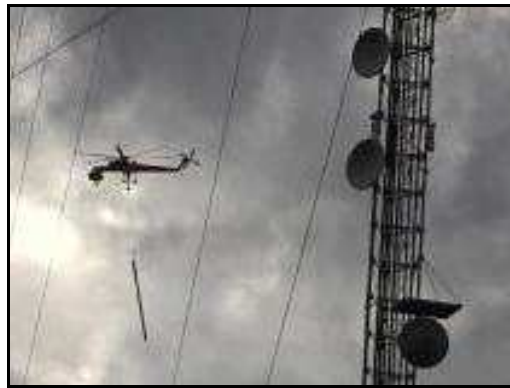
Fig 3 - Old antenna going down! Photos by W4YDY
