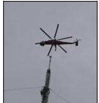
Fig 4 - New Ant installed
