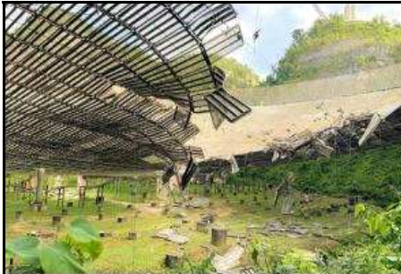
The main collecting dish at Arecibo is among the world's largest single-dish radio telescopes. The reflector disk is 1,000 feet in diameter, 167 feet deep, and covers an area of about 20 acres.
