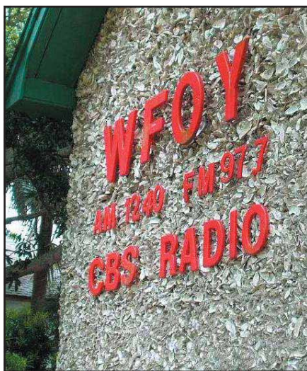
WFOY transmitted from this building for 63 years; those are oyster shells in poured concrete!
