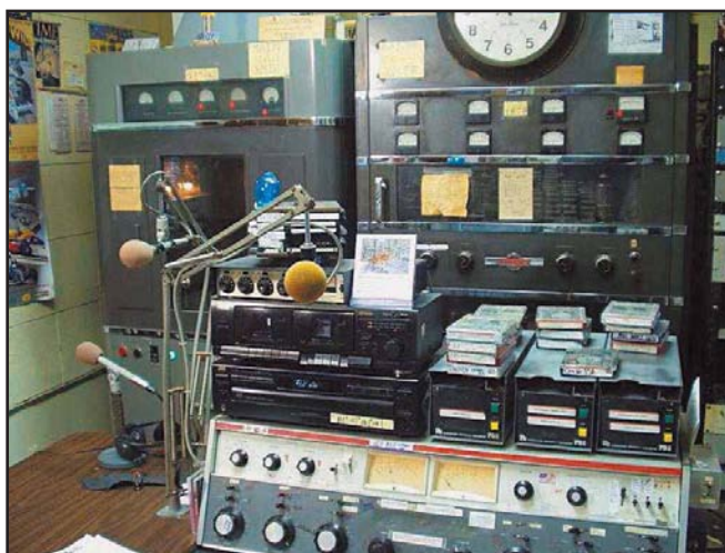
One of the last known pictures of WFOY on the air at its original 1936 location. The Collins 20V-2 is on the left, while the 300-G is to the right.
