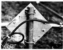
Fig. 10-15 — The boom-to-mast plate.
