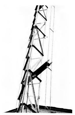
Fig. 13-12 — A board fitted with standoff insulators and clamped to the tower with U bolts keeps open-wire line suitably spaced from a tower. (W4NML.)
