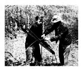
Fig. 14-11 — Proper tension can be placed on the guy wires with the aid of a block-and-tackle system. (Photo by K1THQ)
