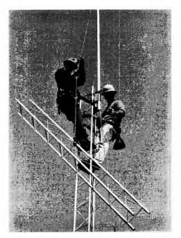
Fig. 14-9 — The assembly of tower sections is made simple when a gin pole is used to lift each one into position. Note that the safety belts of both climbers are fastened below the pole thereby preventing the strap from slipping over the top section. (Photo by K1THQ)
