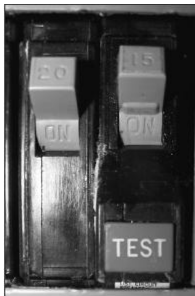
Figure 3.13 — The ground-fault circuit interrupter (GFCI) circuit breaker interrupts current flow when it senses imbalances between the hot and neutral circuits in ac wiring. The imbalance of currents indicates that a shock or other safety hazard exists in wiring supplied by the breaker. Electrical outlets with a built-in GFCI may be found in kitchens, bathrooms, basements, garages and other damp areas.
