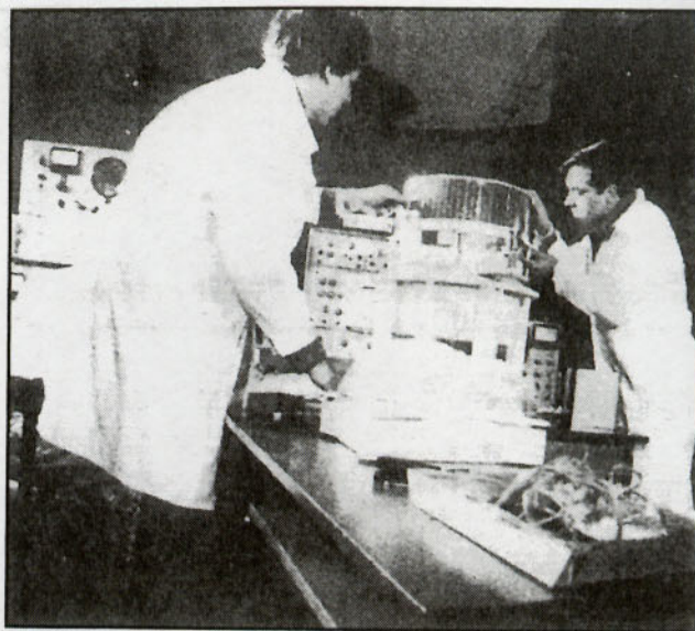
Two technicians assemble the Radio-2 artificial satellite. With Radio-1, this satellite provided communications for more than 700 Amateur Radio operators from 70 countries on all continents. Its communication range was 8000 km (5000 miles). (Photo courtesy Novosti, provided by the Embassy of the USSR)
