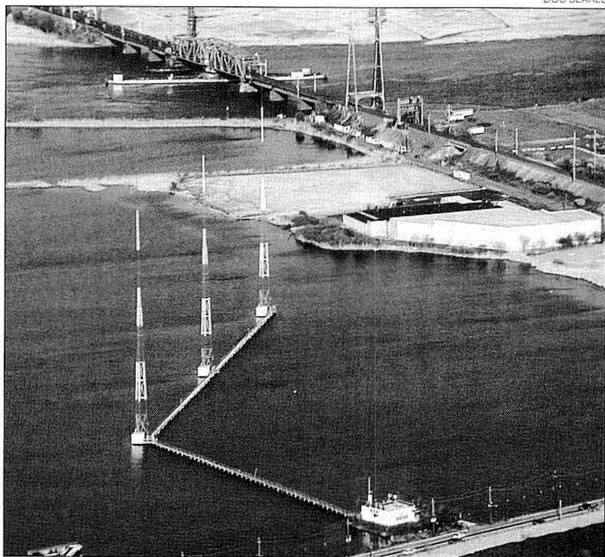
The shared AM antennas of WMCA/WNYC standing in a saltwater tidal marsh in New Jersey. Their massive networks of radial conductors are constantly bathed in saltwater, the ideal environment for a radial ground system.
