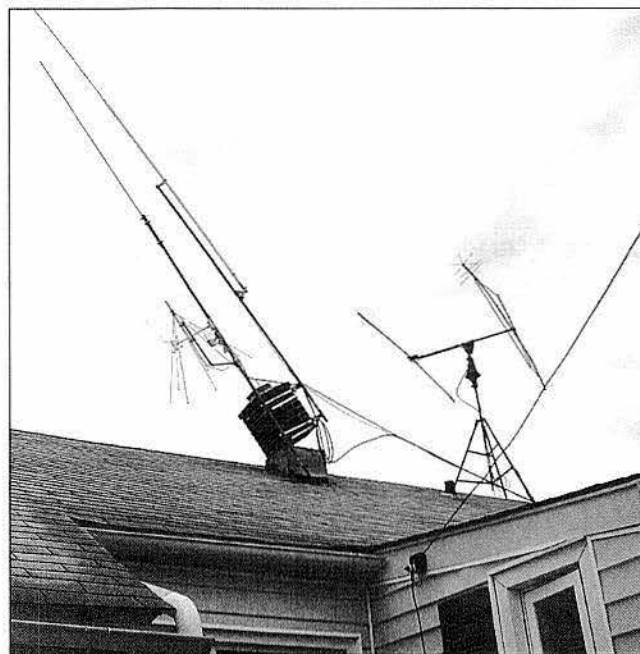
Figure 4.16 — Placing too many antennas and too much wind loading on a chimney can produce catastrophic results!
